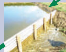
Weeping Wall / Drying Bed
